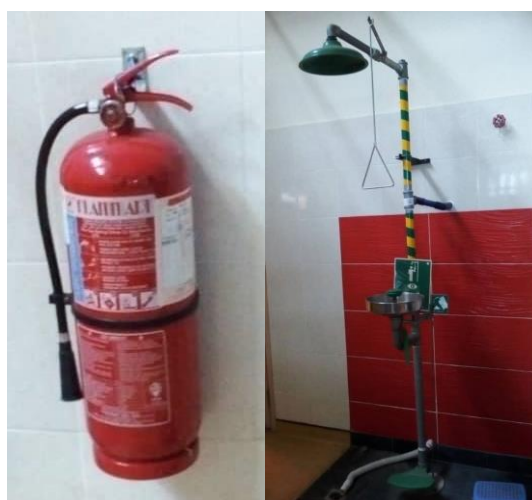
The fire extinguisher, eye wash and safety shower in the Second Year Organic Laboratory
