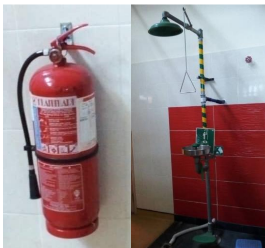
The fire extinguisher, eye wash and safety shower in the First Year Organic Laboratory.
